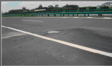
Lag of road maintenance management
